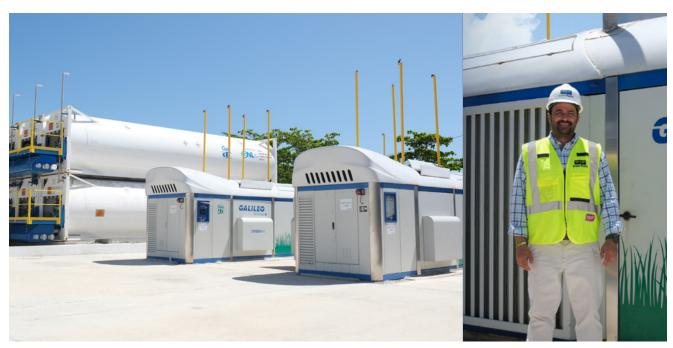
† Two of Galileo's Cryoboxes in operation at a sanitary landfill in Puerto Rico.
